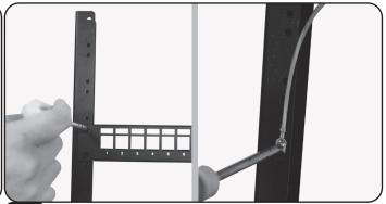
Attach the patch panel and loose end of the grounding wire to the rack.
